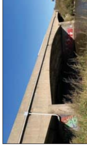
Credit River Bridge
